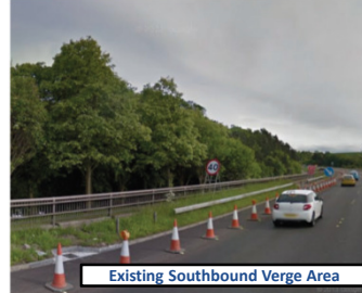
Existing Southbound Verge Area
